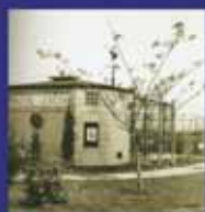
Mike I's new home on LSU's campus in 1937.
