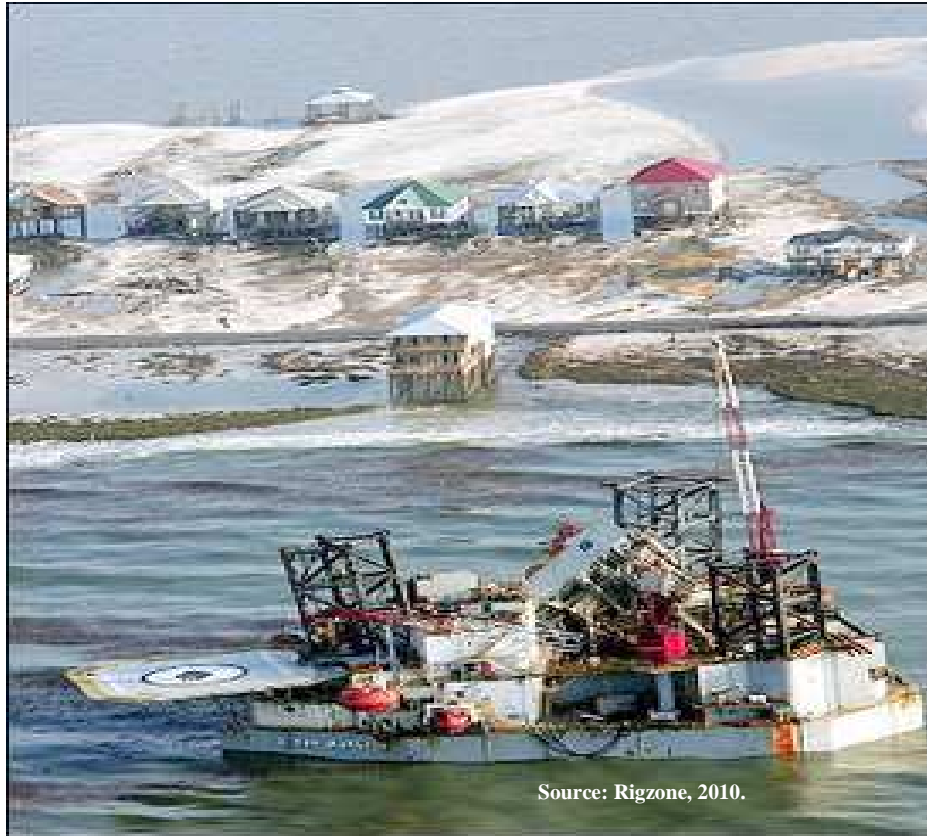
Figure 19. Post-Katrina damage to the Ocean Warwick drilling rig.
