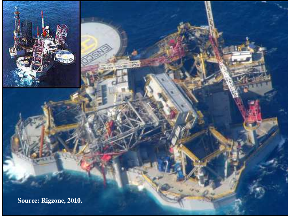
Figure 14. Ensco 64 drilling rig after Hurricane Ivan struck. 21
