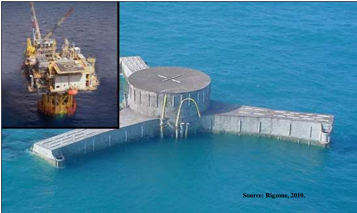
Figure 23. Chevron’s Typhoon Mini-TLP after Hurricane Rita.
