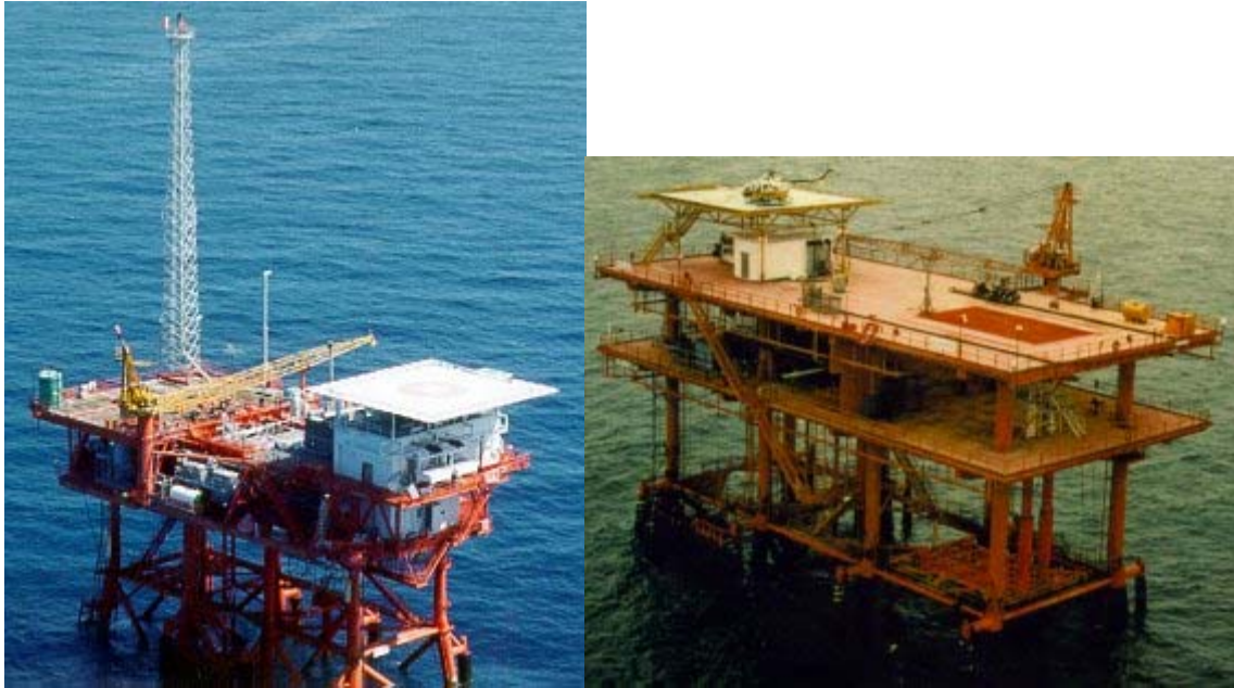
Figure A.4: Fixed Platform Structures.
