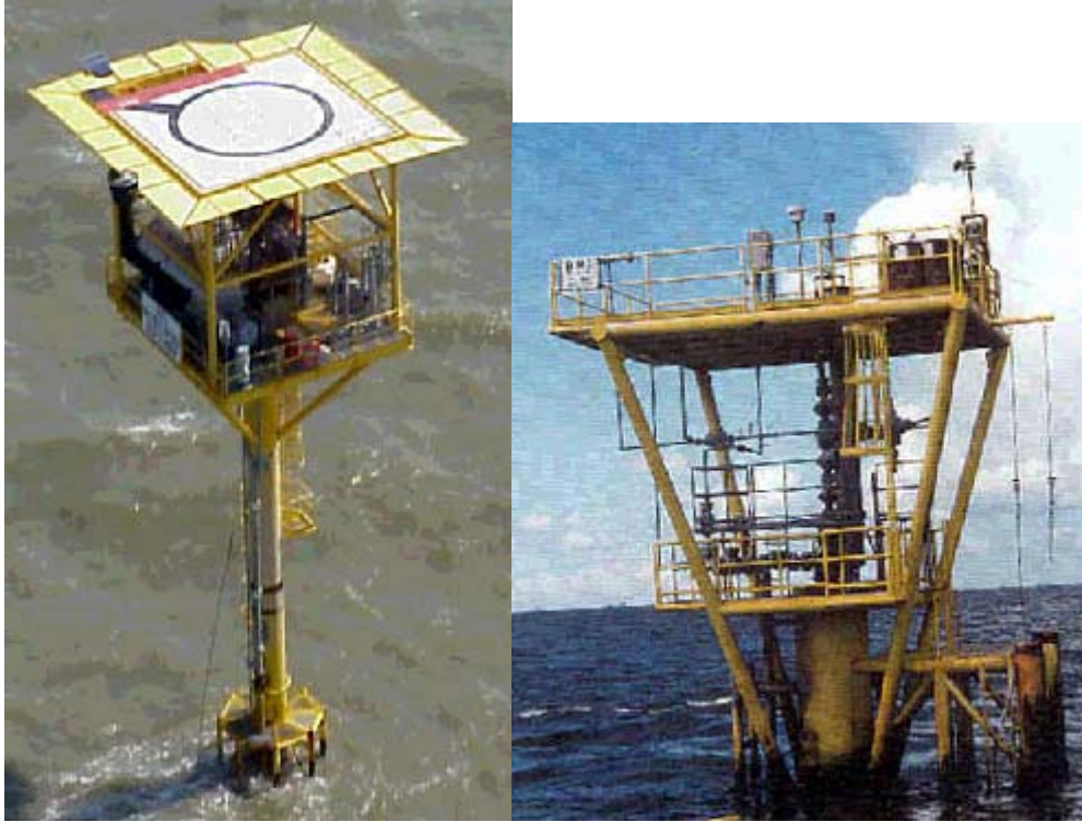
Figure A.2: Caisson Structures.
